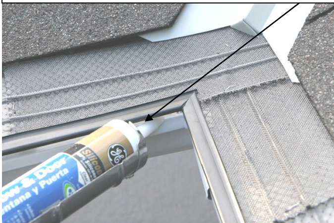
Before you screw U-Channels at inside gutter corner, put a bit of clear silicone caulking between U-Channels and gutter rim (approx. 6" in each direction).
