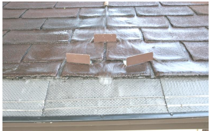
Water-Speed Controllers installed on straight part of asphalt shingle roof. They can be installed in a similar way on any other type of roof.
