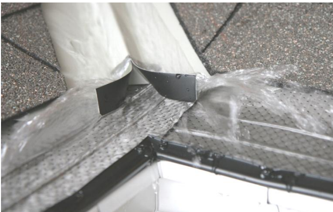
Adjust and re-form the metal strips as needed to spread the water over the largest possible area of IG2™, eliminating overflows and leaks.
